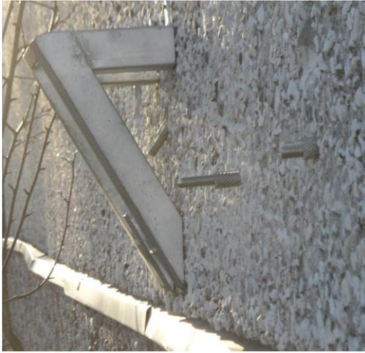
Fig. 4. View of steel frame with anchors.
