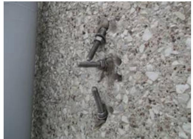
Fig. 6. Anchoring COPY-ECO system and three anchor system.
