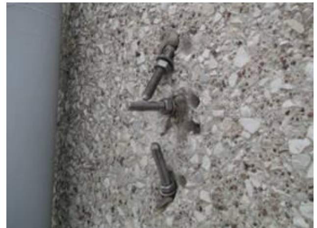
Fig. 6. Anchoring COPY-ECO system and three anchor system.
